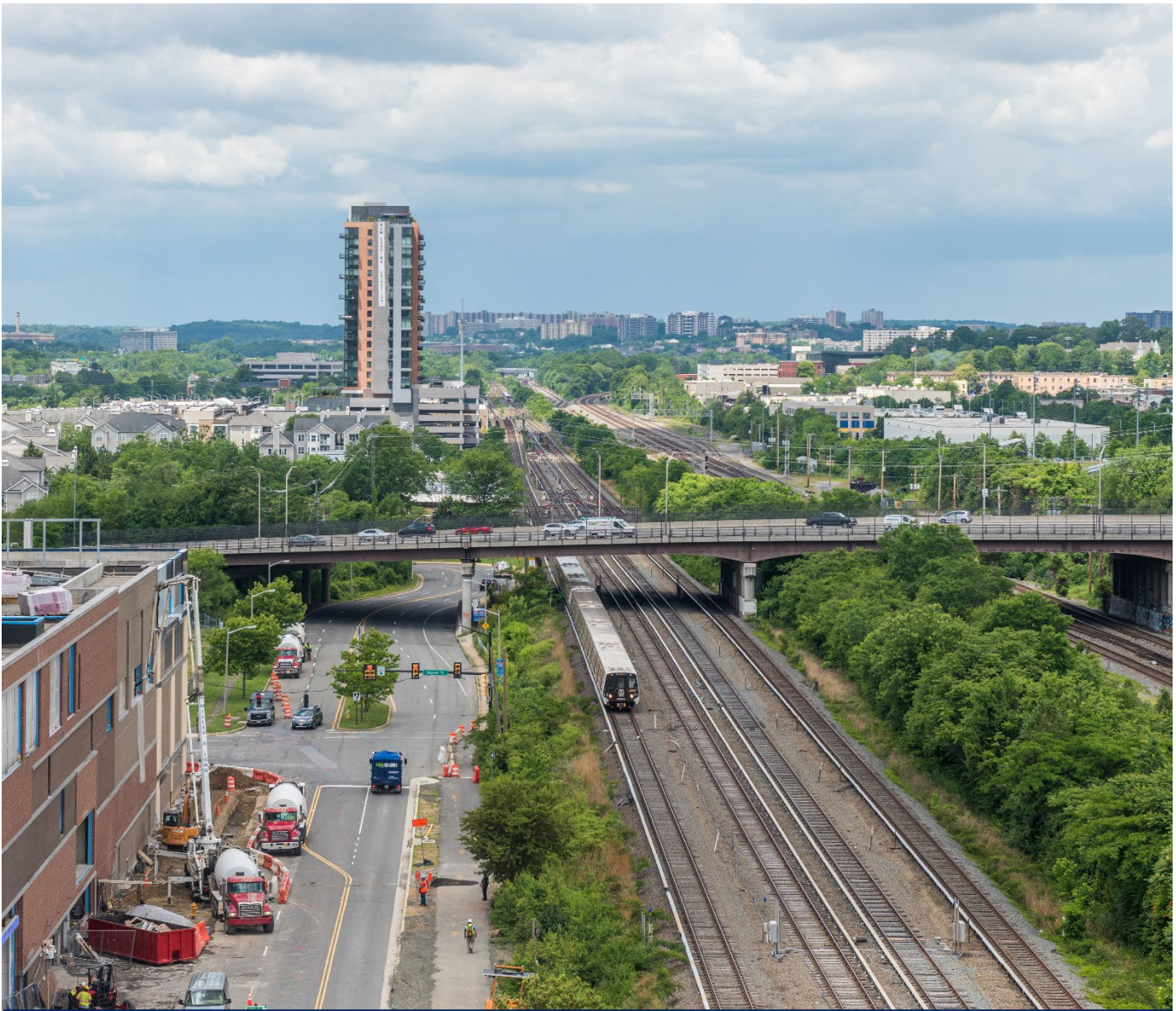
Construction for new Metro office and larger redevelopment near Eisenhower Ave Station
