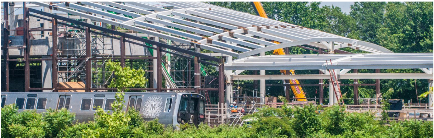
Metrorail train passing by Potomac Yard Station construction
