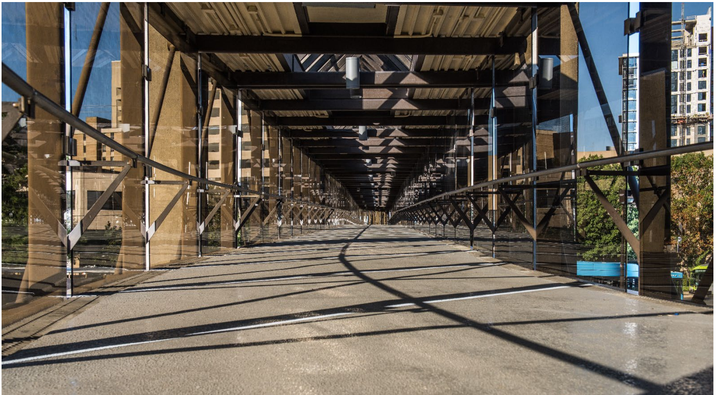
Rockville Station pedestrian bridge
